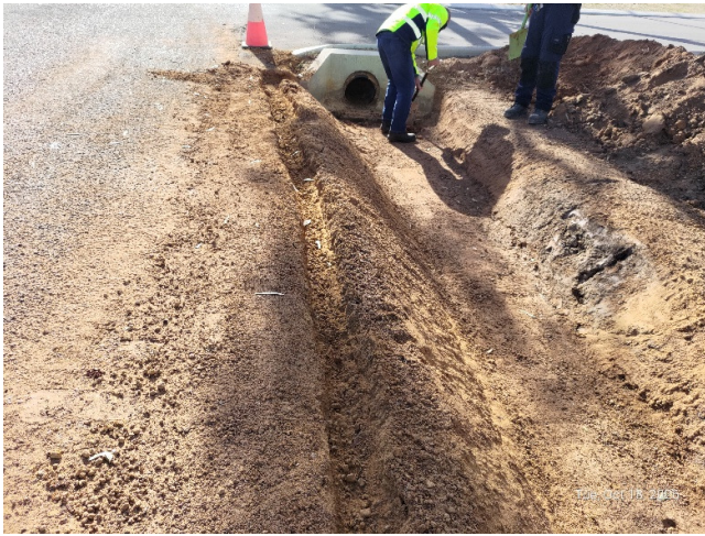
Fig. 5 and 6 Anchor trenches dug out on side slopes along the invert
