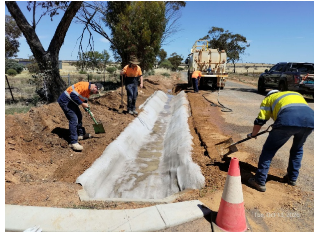
Fig. 19 Once the cementcrete composite blanket was hydrated, it is backfilled with road base material
