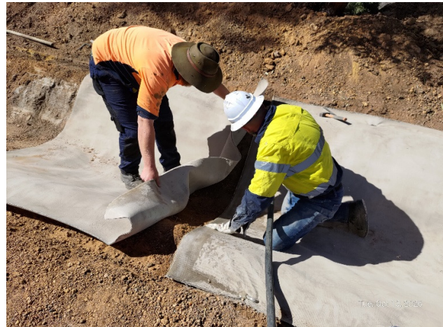
Fig. 9 Overlapping the layers by at least 100mm
