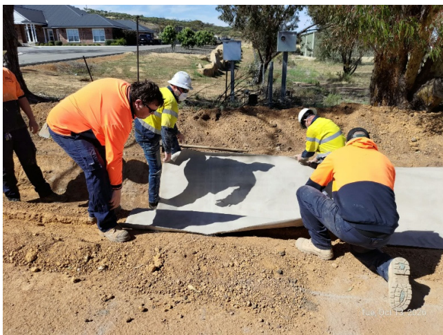
Fig. 10 Adjusting cementcrete composite blanket with hand repositioning
