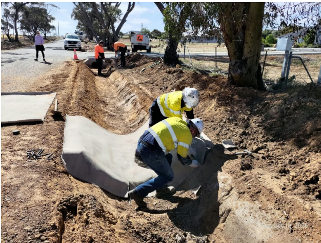
Fig. 11 & 12 First layer of the cementcrete composite blanket is tucked into the anchor trench
