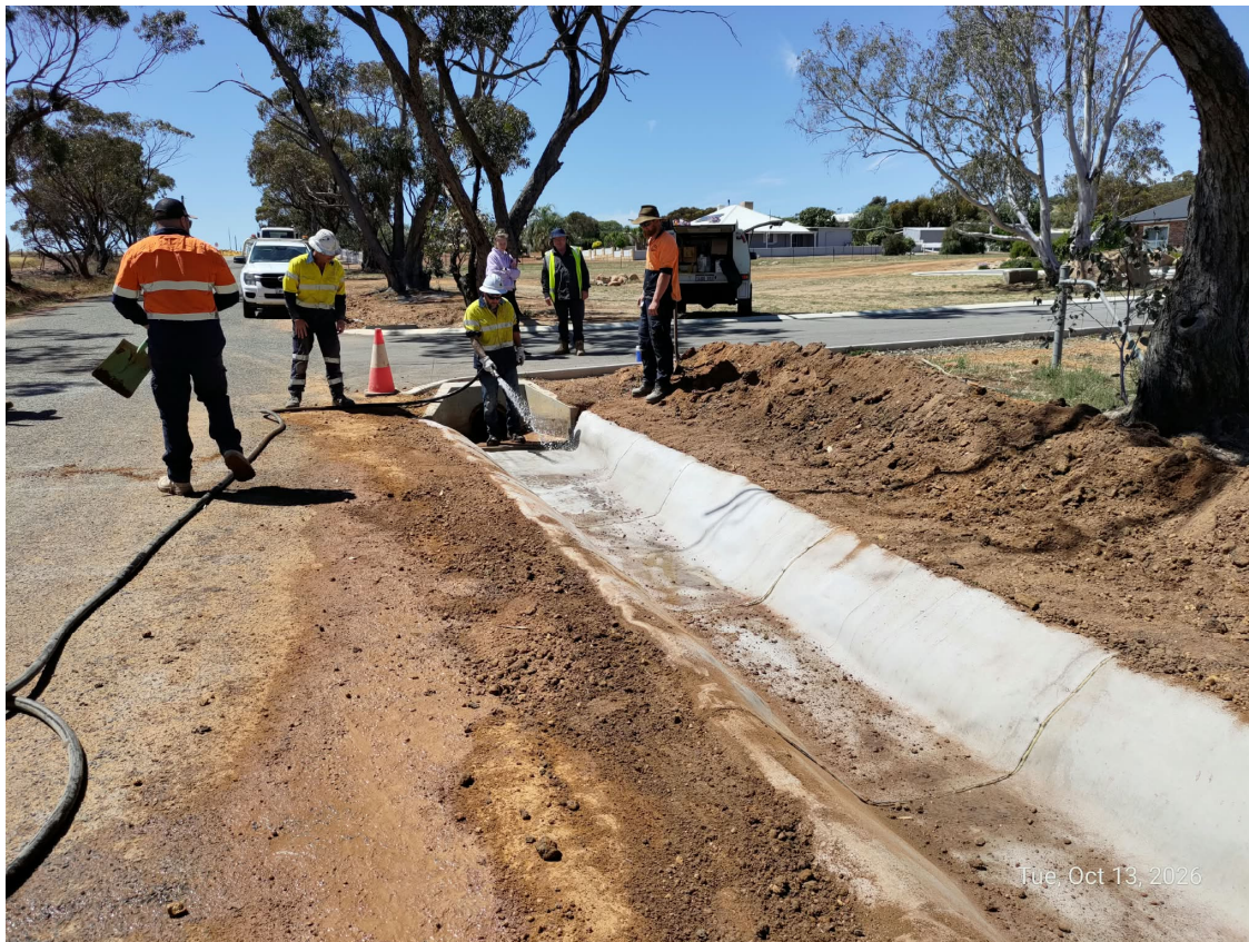
Fig. 21 The cementcrete composite blanket is hydrated with water after joining, fixing and backfilling
