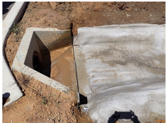
Fig. 13 & 14 Last layer of the cementcrete composite blanket is tucked into the anchor trench
