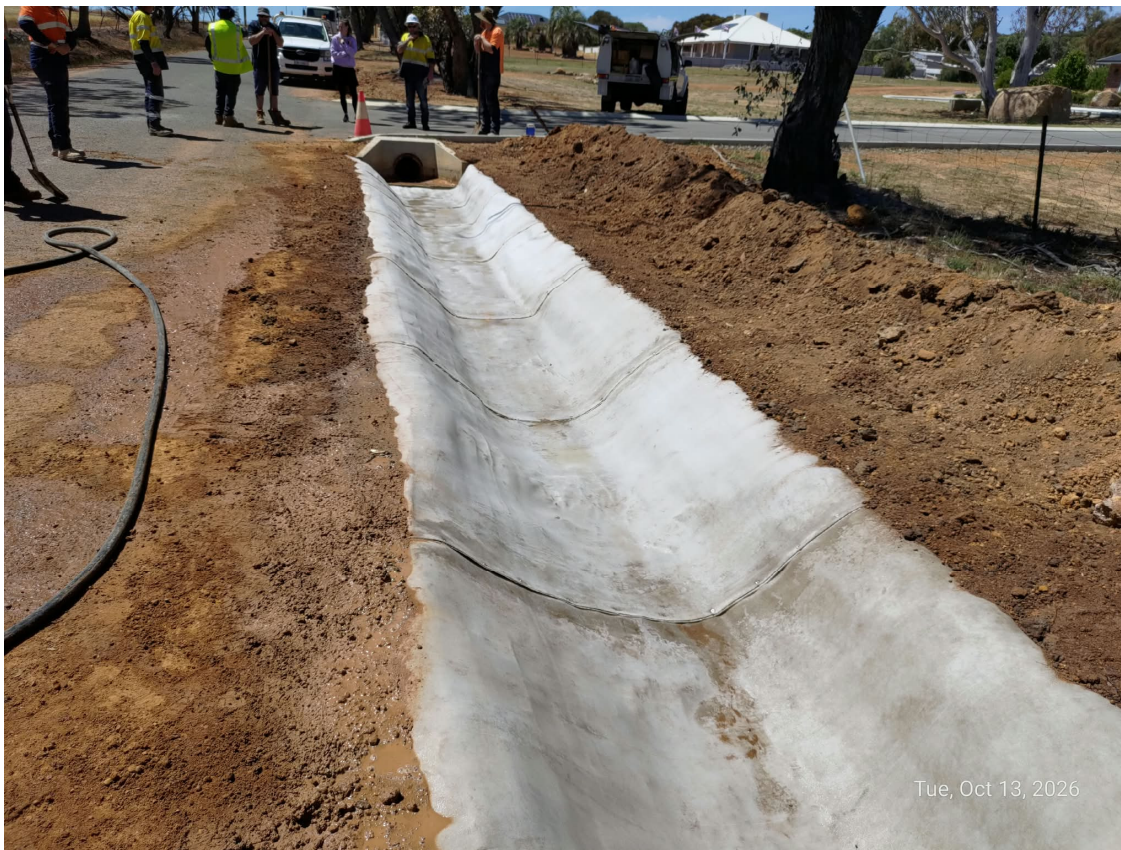
Fig. 22 The finishing layout of cementcrete composite blanket on roadside drainage channel
