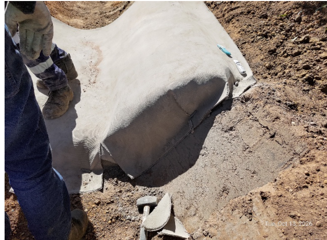
Fig. 11 & 12 First layer of the cementcrete composite blanket is tucked into the anchor trench
