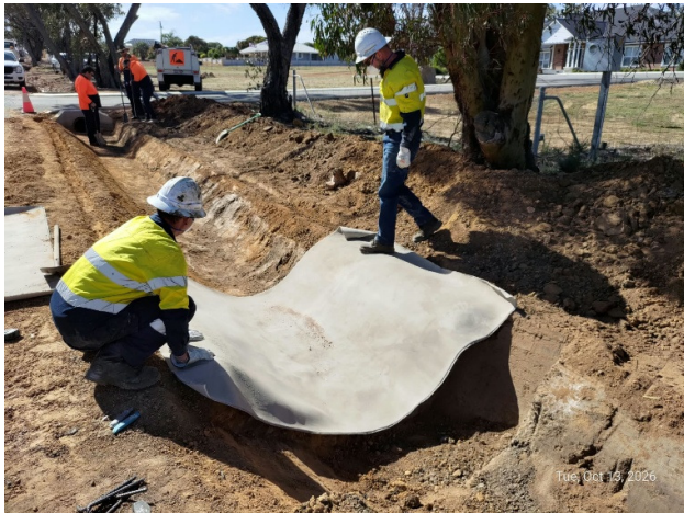
Fig. 8 Cementcrete composite blanket lay by begin at the downstream end of channel
