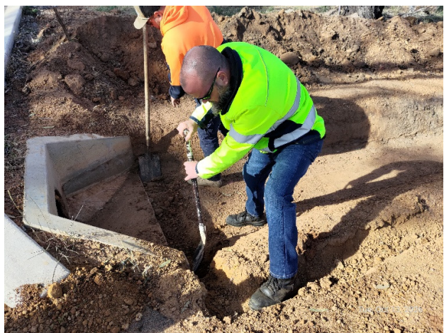
Fig. 13 & 14 Last layer of the cementcrete composite blanket is tucked into the anchor trench
