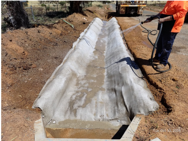
Fig. 18 The cementcrete composite blanket is hydrated with water
